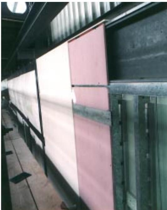
*A close up of the 15mm and 10mm boards being fixed*
