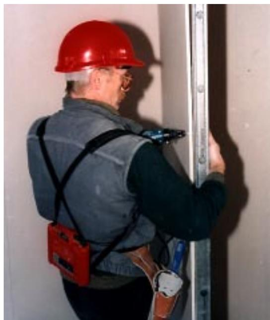
*Battery-powered hand tools for screw-fixing wallboard to the metal frame*
