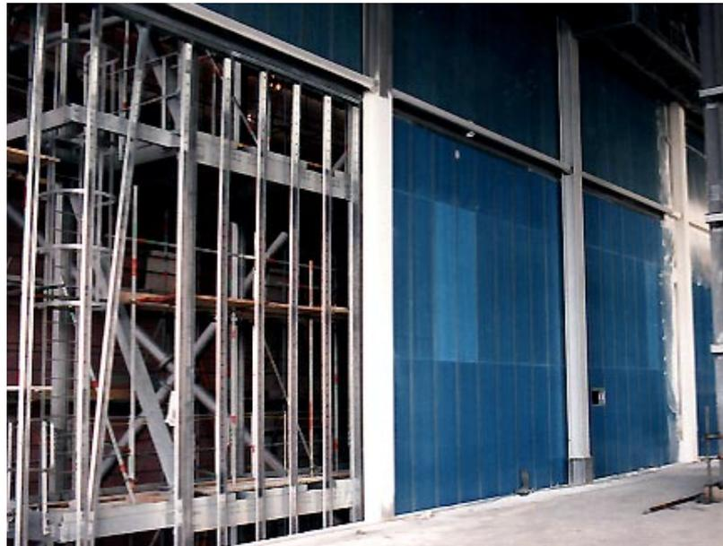
*The vapour check core board being fixed from the scaffolding behind*
