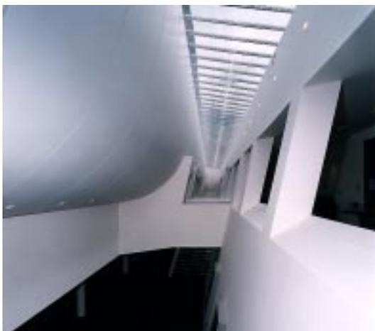
*An elliptical barrel ceiling formed from gypsum wallboard*
