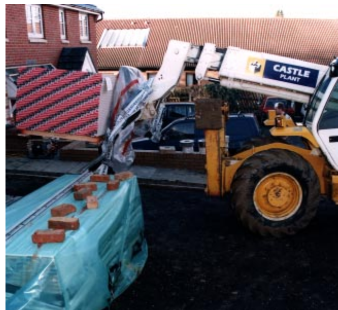
Avoiding direct waste by correct handling and storage
