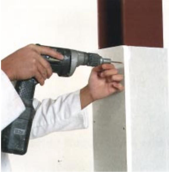
*Glass reinforced gypsum board being used to provide time protection to structural steelwork*
